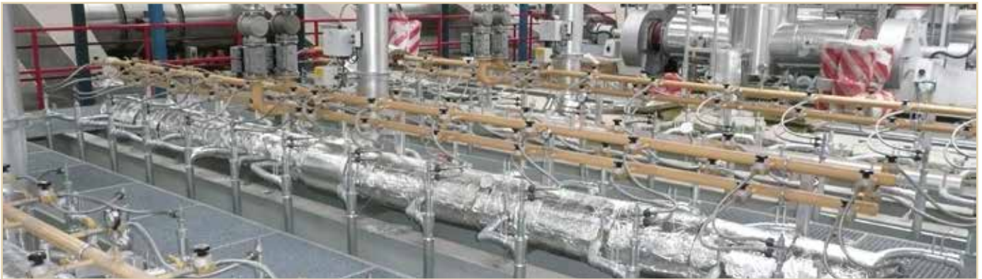
Reduction group with extra gas supply for reduced firing
