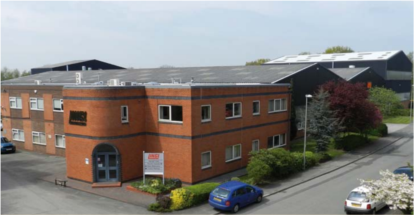
Aerial View of LINGL LUK Premises
